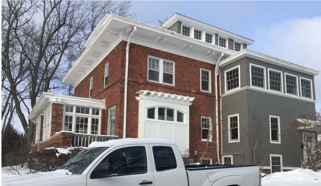
Photo 1 – View of the building from the southside lot line
